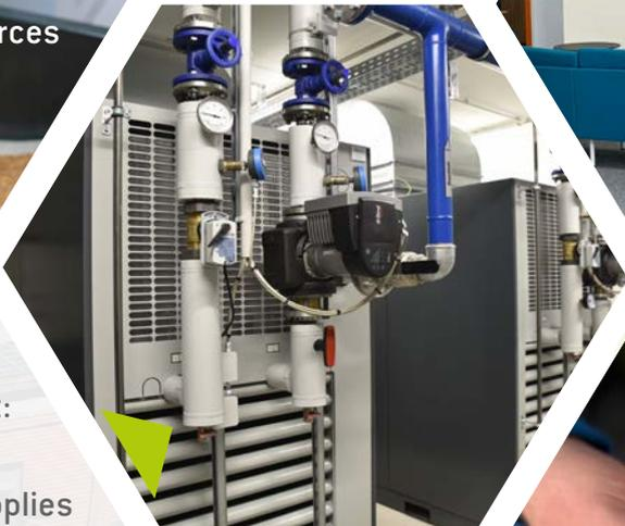
... heating with waste heat: The waste heat compressor supplies the new buildings with heat generated from compressed air in production.
